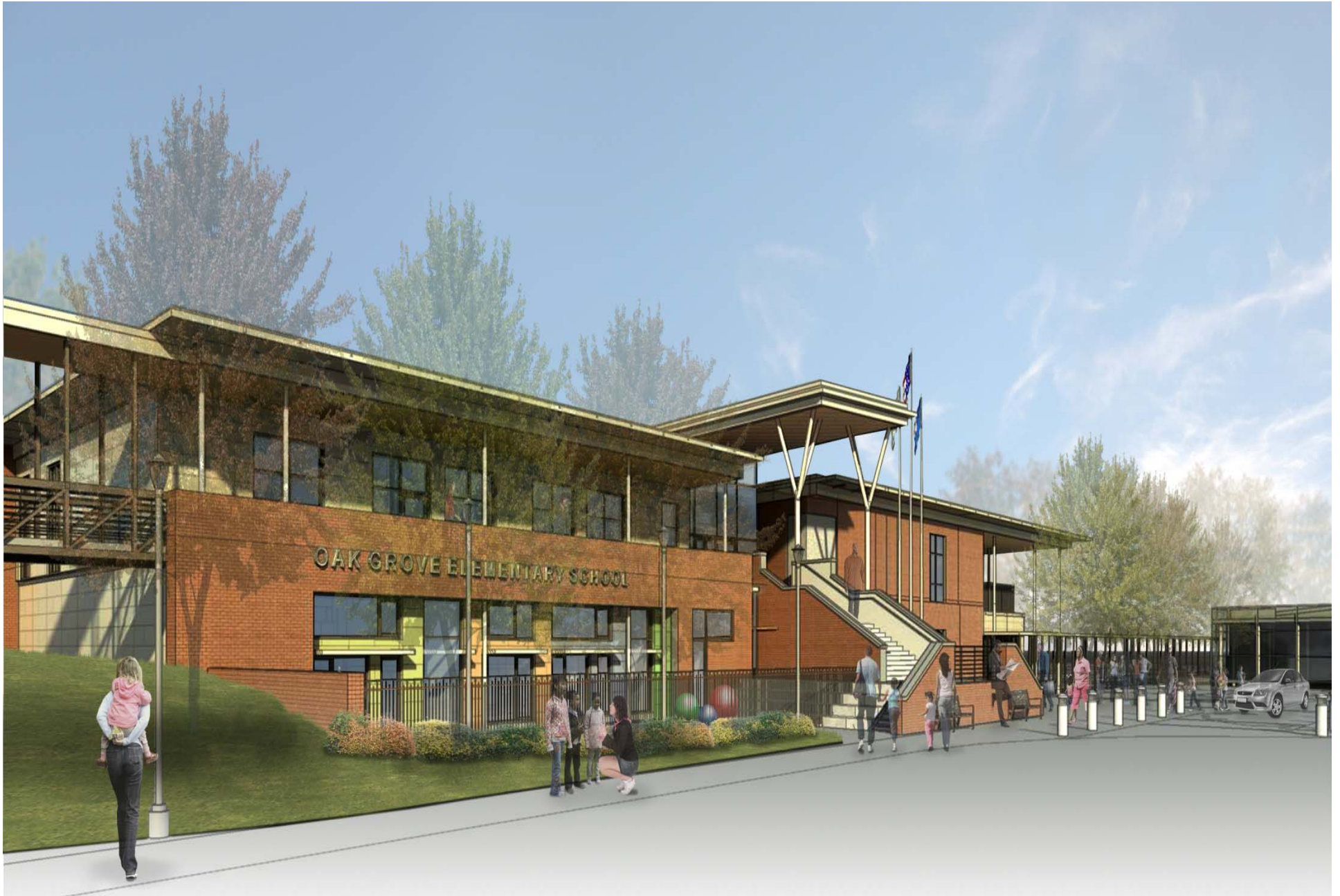
Oak Grove Elementary School - Entry
